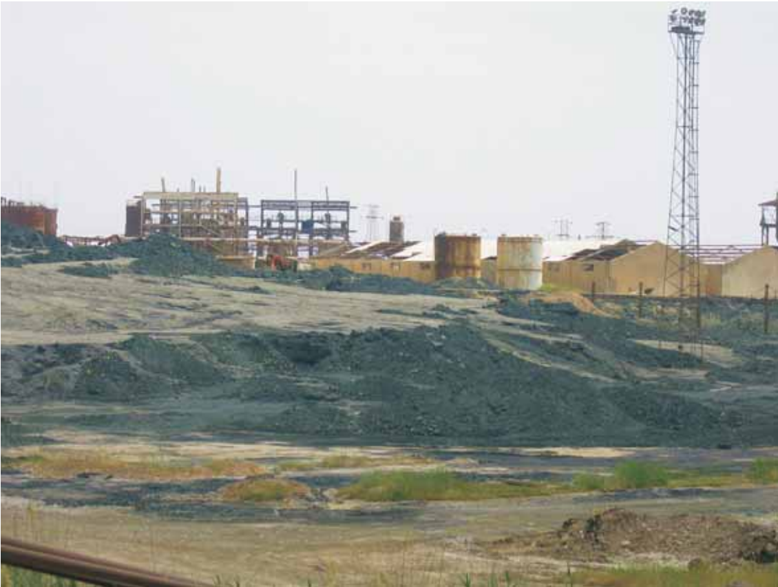
Asphalt containing waste piles in front of the sulphur purification plant
