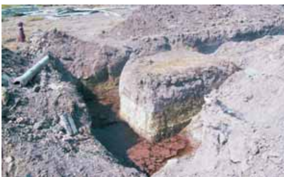
Site entrance at Al Qadissiya showing perched groundwater at 2 m depth
