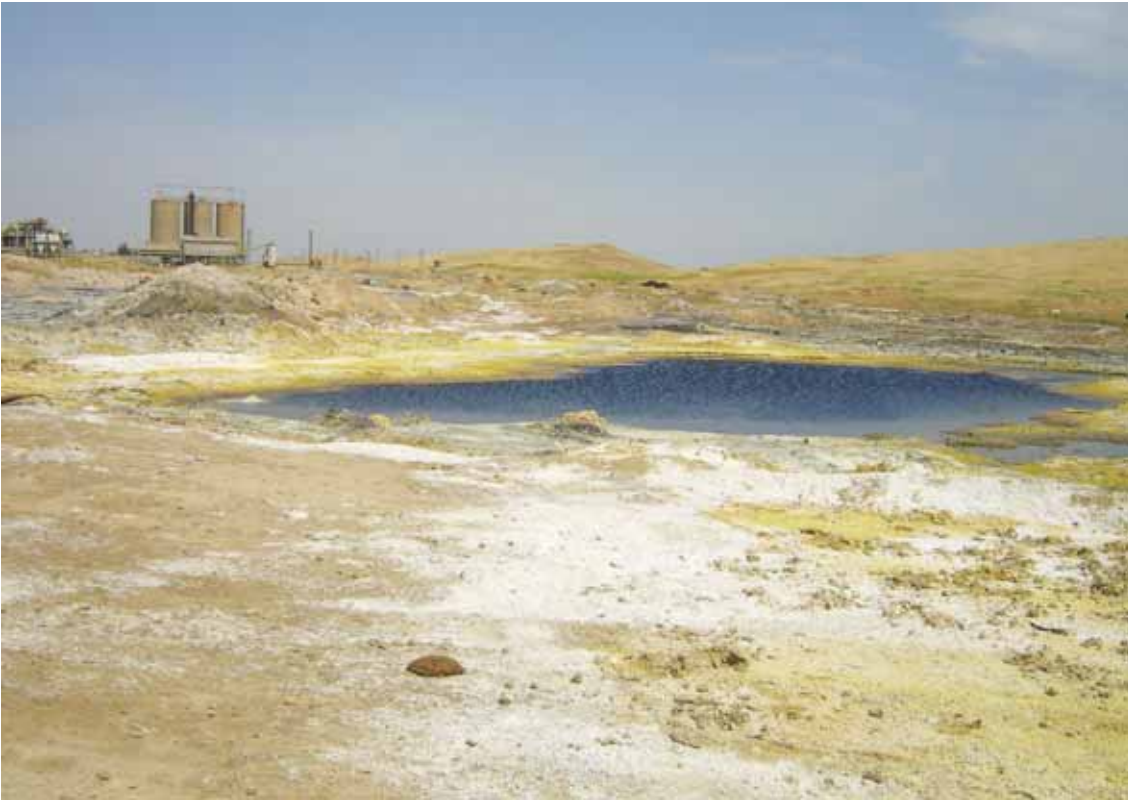
Drainage ponds close to the acid plant contain dilute sulphuric acid
