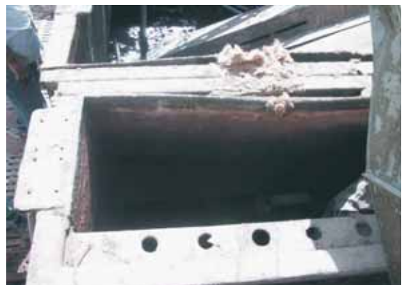
Chemical wash tanks still containing spent liquor
