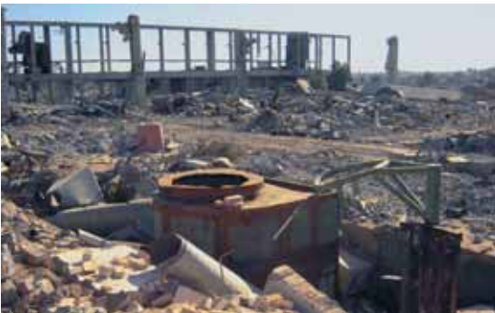
Site after uncontrolled demolition with chemicals dumped in place
