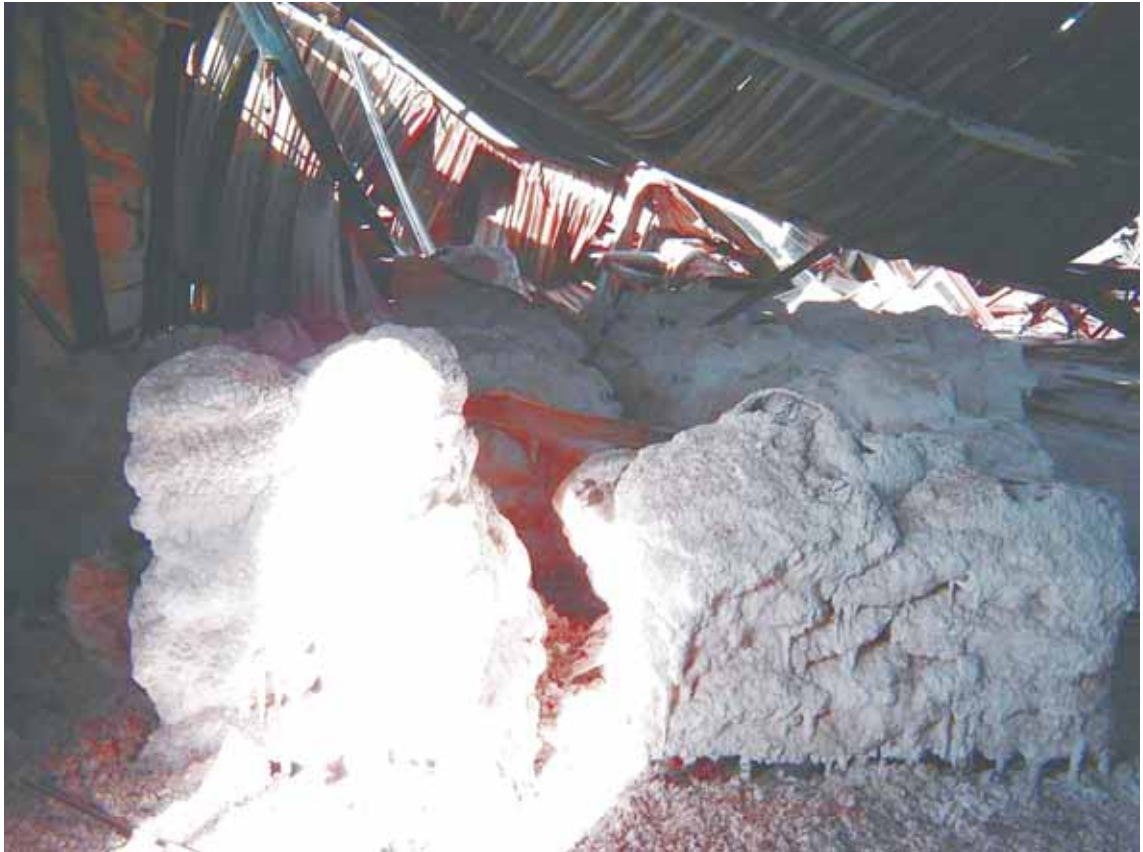
Damaged stocks of sodium hydroxide remain inside the burnt out warehouses
