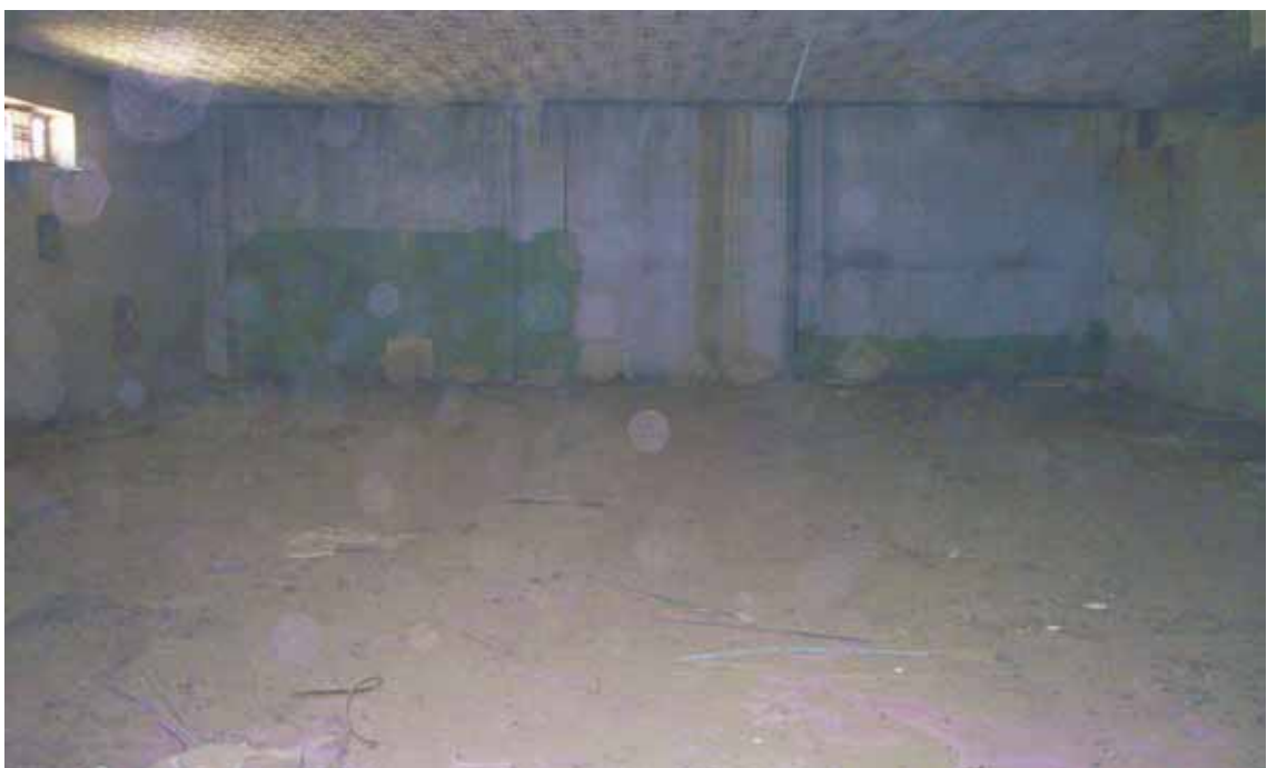
The floor, walls and ceiling of the warehouse need decontamination to allow it to be used again
