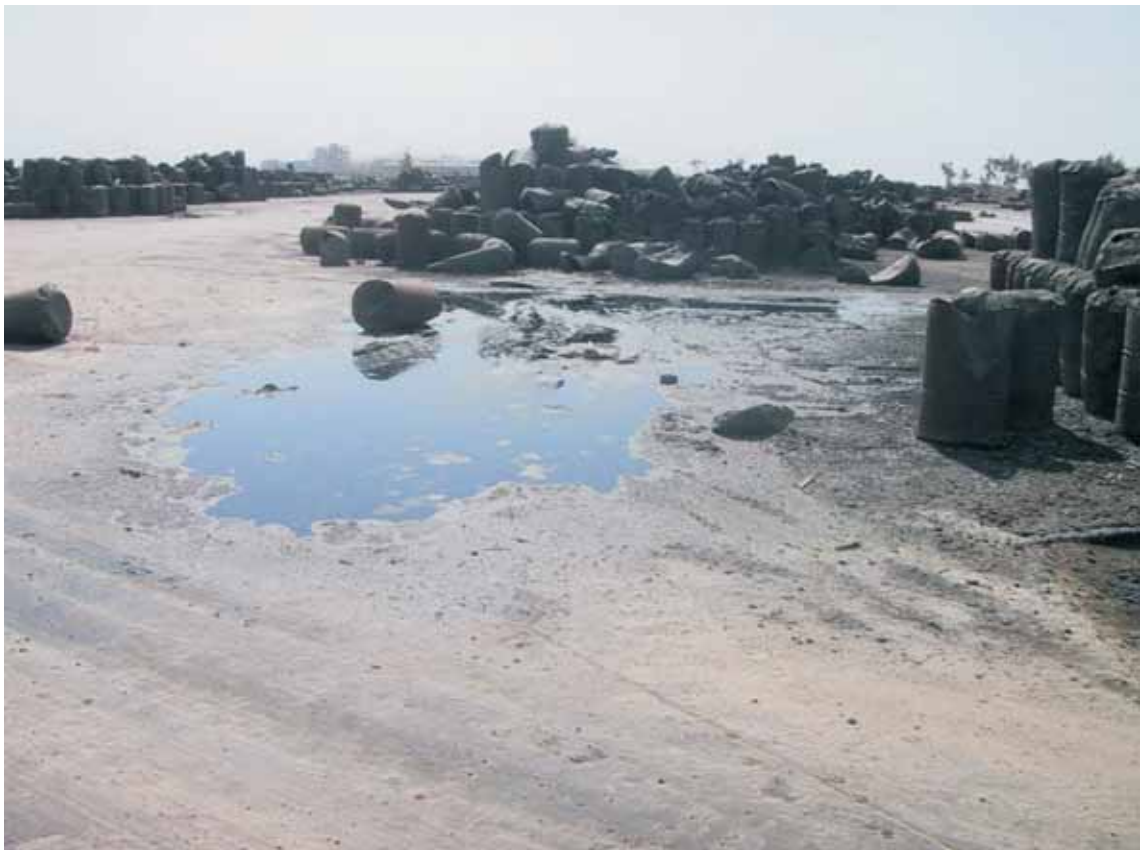
Both the spilled chemicals and the damaged drums will need to be removed
