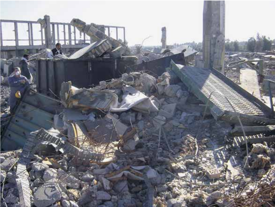
Uncontrolled demolition of Al Qadissiya
